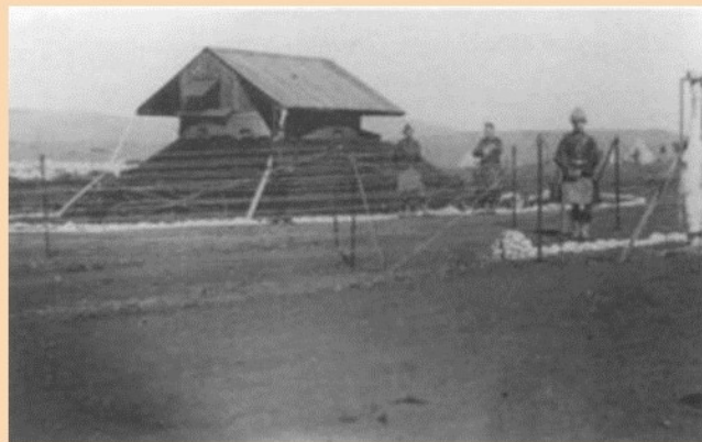
A blockhouse, made of two skins of corrugated iron nailed onto a wooden frame, situated two miles east of Pretoria, June 1902 (Photo: SANMMH)
